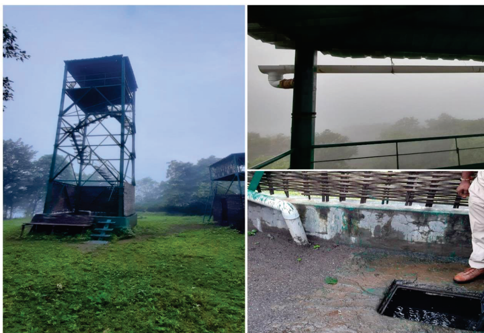
Photograph 4.4: Rain water harvesting structure at Bardipada Range of Purna Sanctuary
